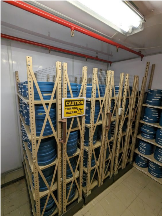
Internal of current Nitrate Vault showing storage system, fire sprinklers and spark proof lights.
