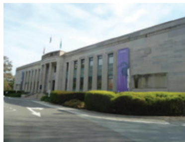
Figure 37: Main Façade – Sandstone Faced Fluted Panels (EMAA 2018)
