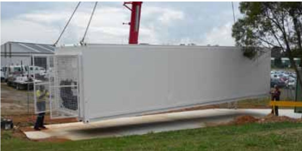
Installation of a new nitrate-compatible container at the NFSA's nitrate site in Mitchell ACT
