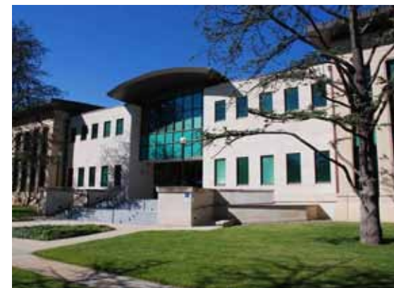
NFSA annex, Liversidge St
